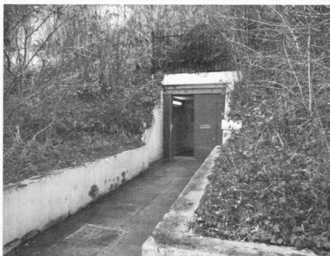
The main entrance to the tunnel complex.
